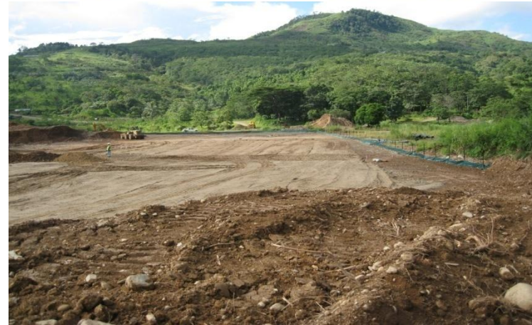
Operations village site clearing commenced
