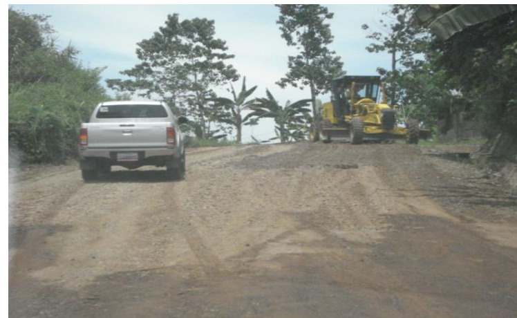
Re-sheeting of access road underway
