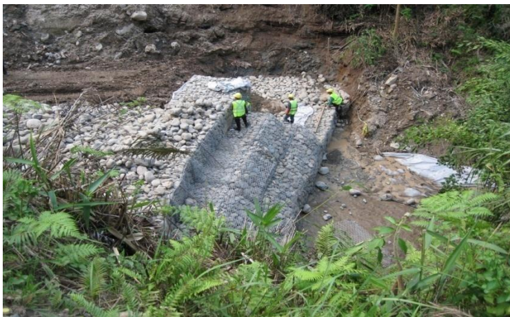
Gabion baskets at access road drain
