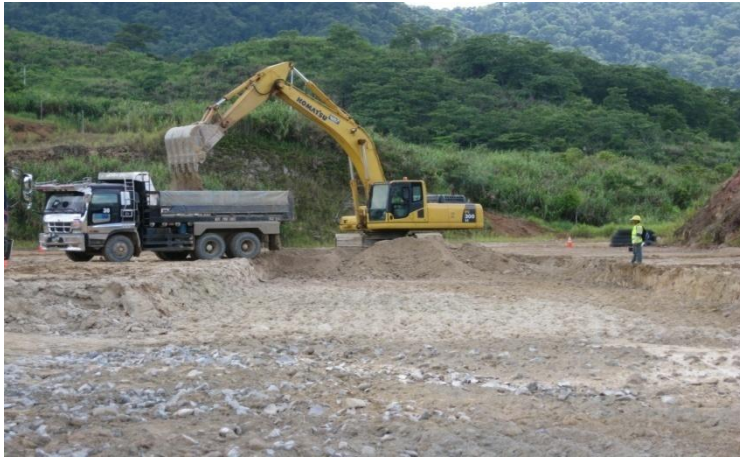
Final earthworks underway at process plant site
