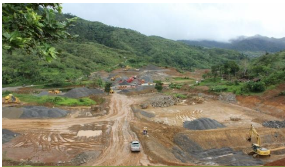
TSF crusher lay down area
