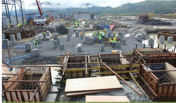
Tailings thickener formworks
