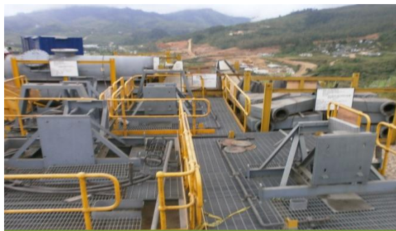
Equipment on site
