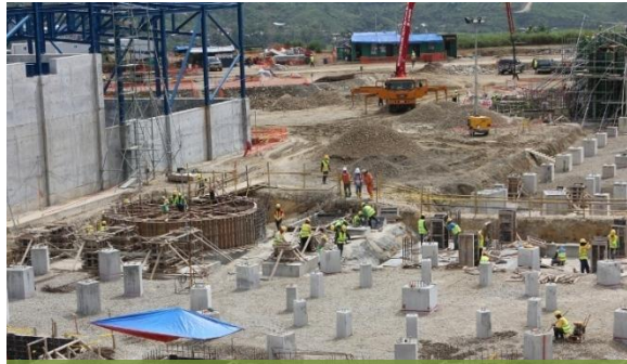
Tank base concentrate handling area
