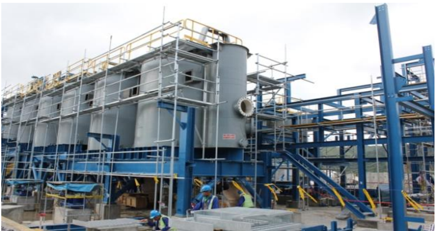
Figure 2: Flotation cells structural and mechanical installation, June 2012
