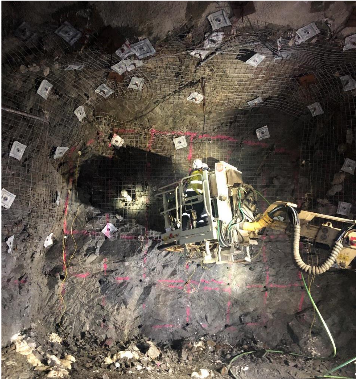
Figure 1 – First Underground Cut at Didipio
